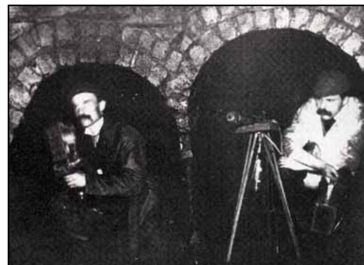
Figure 4.2: Carnelley and Haldane (right) in the Intercept Sewer in Dundee. (Courtesy of Richard Haldane MBE.)
